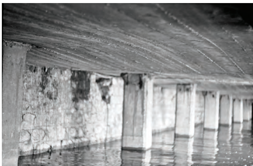
Figure 11. The remains of the fortress pier, 1993. Author's photo, after Şlapac 2024, fig. 122.
